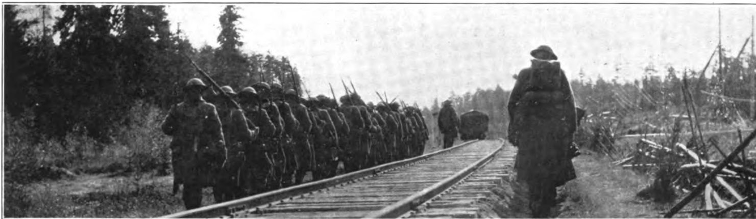
Forward to Hold Bridge at 458.
