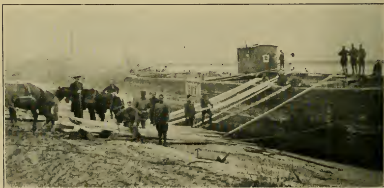
310th Engineers at Beresnik
